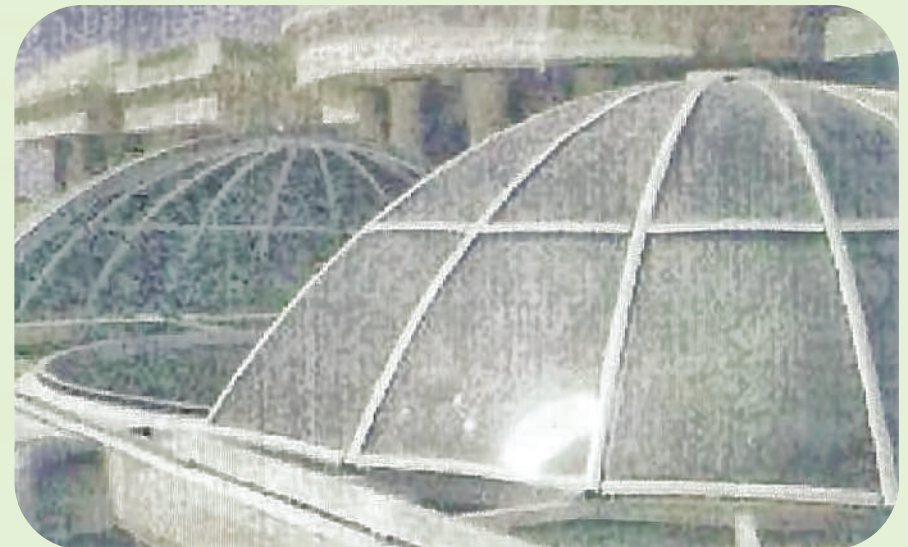
Arched skylight cover Duryea mall. Riyadh.
