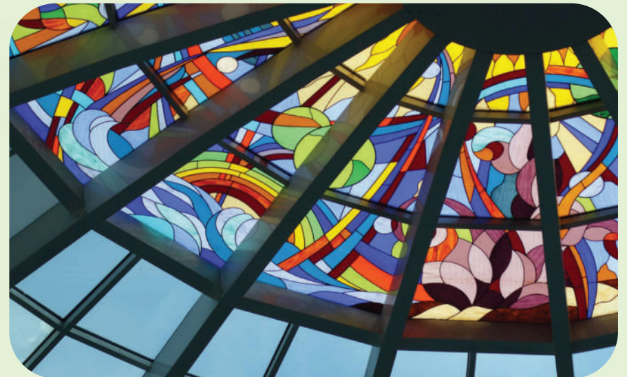
The glass on space frame (spider system dome)
